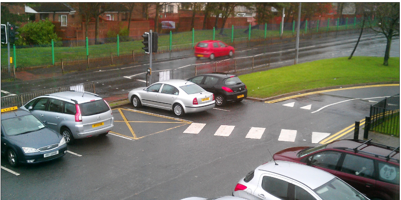
New speed ramp and pedestrian footway
